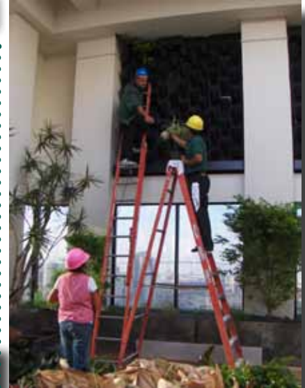
Workers at Greenscaped Building's Procopio Living Wall
